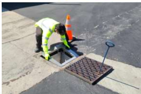
Figure 10 - Grate Inlet Filter (no access window) Being Installed.
