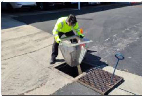
Figure 9 - Grate Inlet Filter (no access window) Being Installed.
