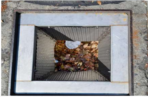
Figure 13 - Grate Inlet Filter (no access window) Prior to Maintenance.
