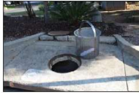
Figure 16 - Curb Inlet Filter Basket Being Installed.
