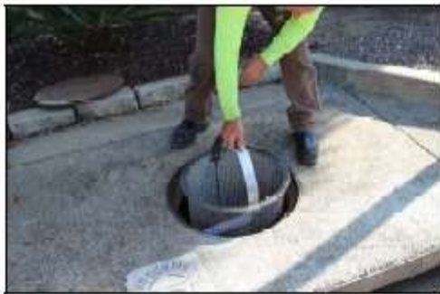
Figure 17 - Curb Inlet Filter Basket Being Installed.
