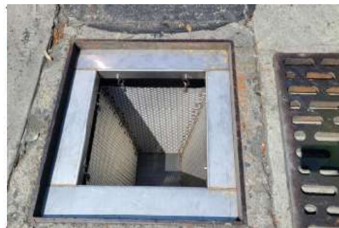
Figure 11 - Grate Inlet Filter (no access window) installed.
