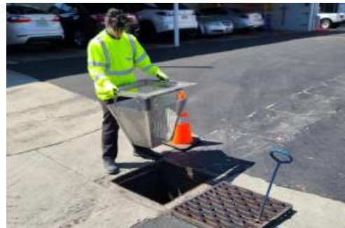
Figure 8 - Grate Inlet Filter (no access window) Being Installed.
