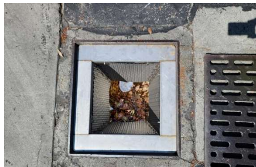
Figure 12 - Grate Inlet Filter (no access window) Prior to Maintenance.
