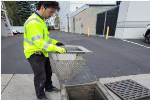
Figure 7 - Grate Inlet Filter (no access window) Prior to Installation.
