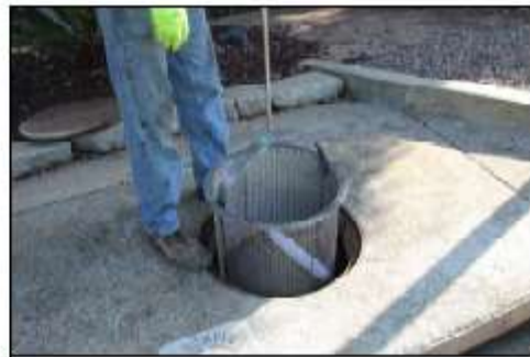
Figure 18 - Curb Inlet Filter Basket Being Installed.
