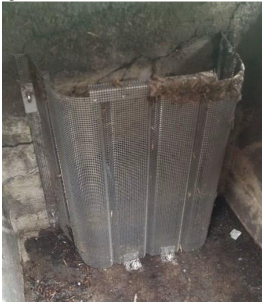
Figure 4 – Connector Pipe Screen Installed (U-Shaped)
