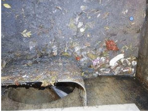
Figure 6 – CPS Before Maintenance (U-Shaped)
