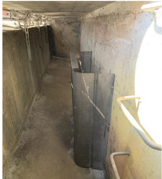
Figure 5 – Connector Pipe Screen Installed (U-Shaped)
