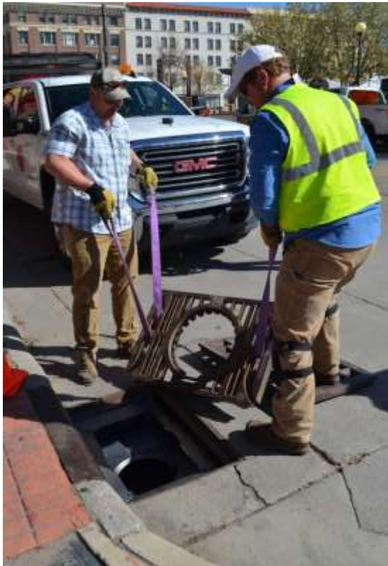
Image 12 - Installation of an optional OGB grate for a DIF-C
