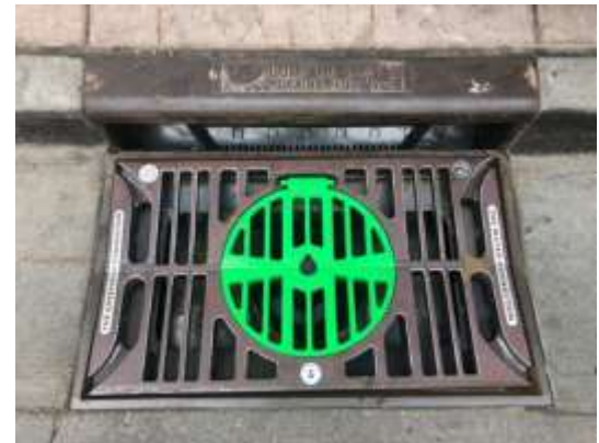
Image 5 - Installed DIF-C with diverter screen and optional OGB grate (access hatch closed)
