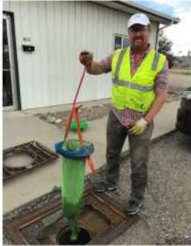
Image 1 - Mundus Bag® removal with storm grate removed
