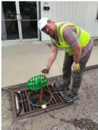
Image 7 - Mundus Bag® removal thru the OGB hinged access hatch
