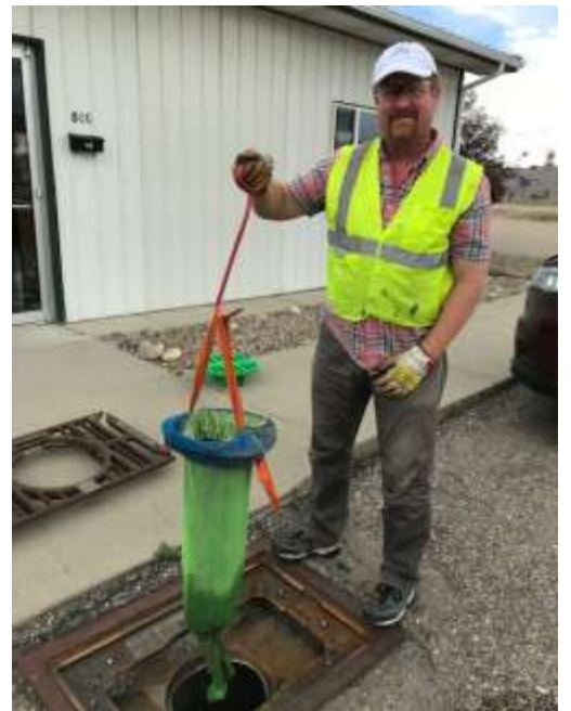
Image 9 - Demonstrating Mundus Bag removal for a DIF
