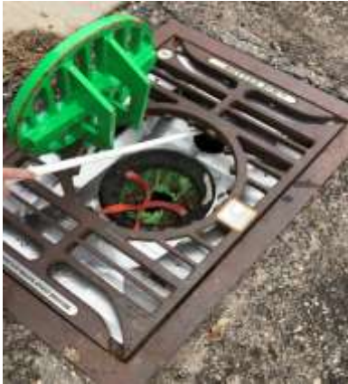
Image 10 – Opening the sample port through the optional OGB grate with access hatch in locked open position and Mundus Bag installed
