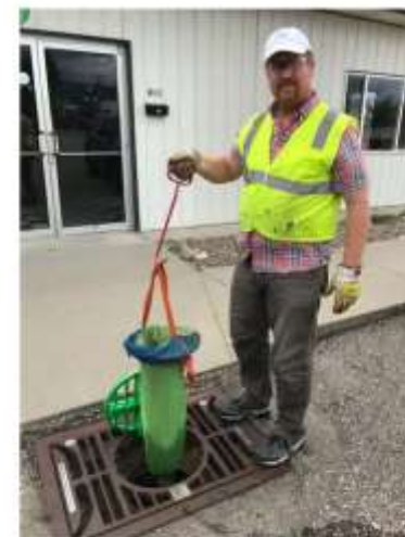
Image 8 - Mundus Bag® removal thru the OGB hinged access hatch
