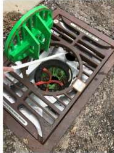
Image 10 – Opening the sample port through the optional OGB access grate.
