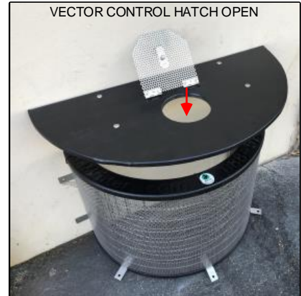
VECTOR CONTROL HATCH OPEN
