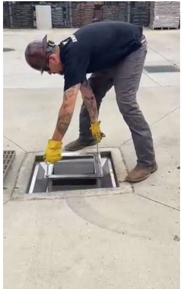
Figure 27 Example of installing the stainless-steel basket within the stainless-steel basket option in a grated inlet (Configuration 1)
