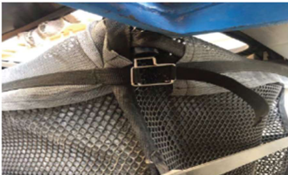
Image of correct liner installation, with fastener attached to the appropriate buckle with no obstruction of LittaTrap™ bypass
