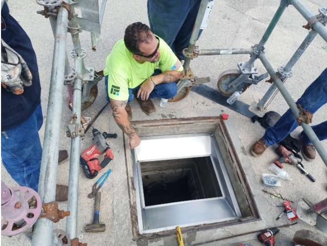
Figure 26 Example of a stainless-steel flange installation on a grate inlet (configuration 1)
