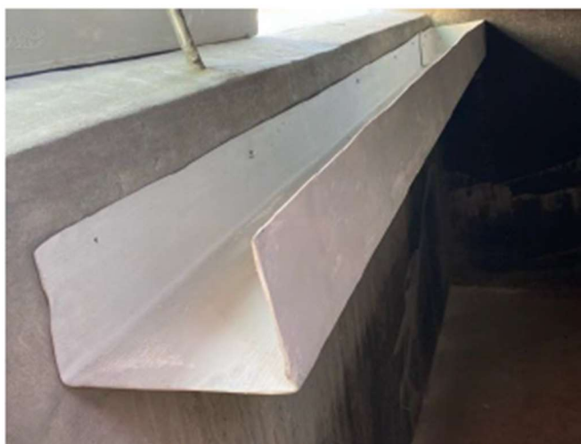
Trough with end cap installed attached to the wall.
