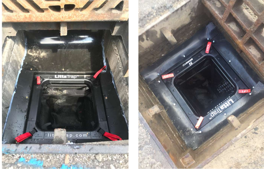
Figure 16 Photos of seal kits surrounding Enviropod® LittaTrap™FC
