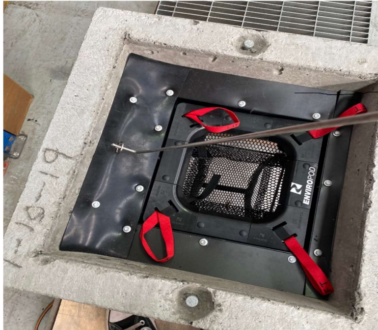
Figure 35: Enviropod® Littatrap™ FC with Vector Inspection seal in closed position. The position and operation is the same for grated inlet catchbasins (Configuration 1), manhole catchbasins (Configuration 2) and combination inlet catchbasins (Configuration 3). Curb inlet configuration 4a and 4b do not require a vector port as they can be inspected via the manhole or inlet.
