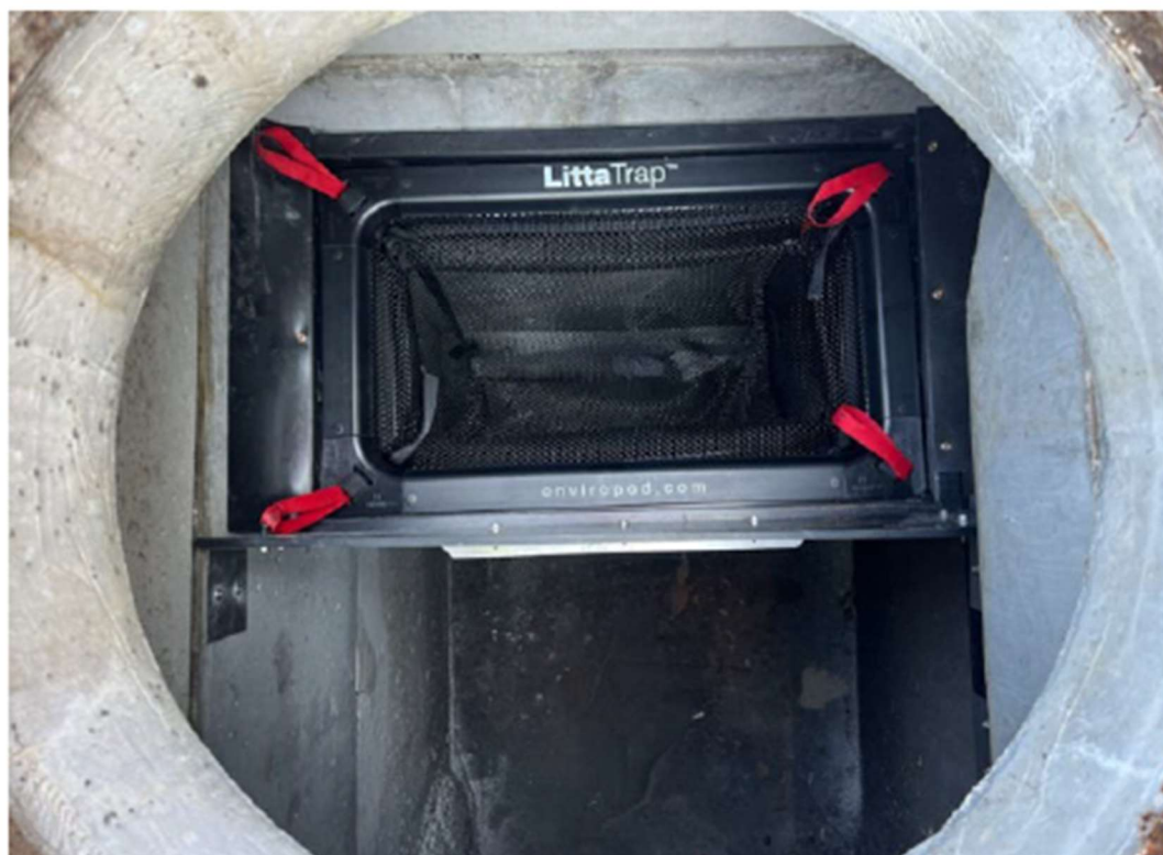
Finished installation with the LittaTrap basket placed in the catch basin.
