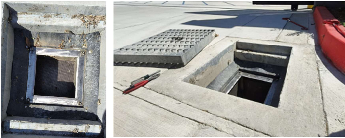
Figure 19 EnviroPod® LittaTrap™ FC stainless steel basket installation (Configuration 1)
