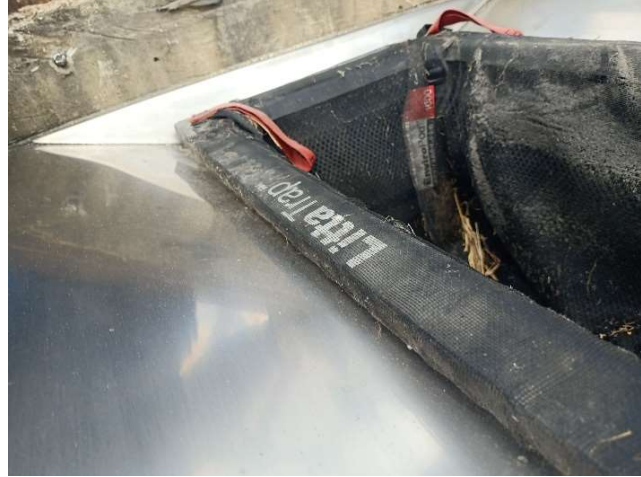
Figure 26 Example of a stainless-steel flange installation on a grate inlet (configuration 1)
