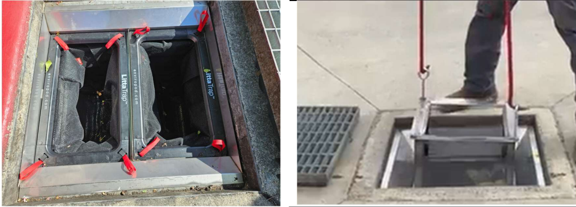
Figure 20 Enviropod® LittaTrap™ FC grated inlet (Configuration 1) installed with a stainless-steel flange (left) and a stainless steel basket being installed on a stainless-steel flange (right).
