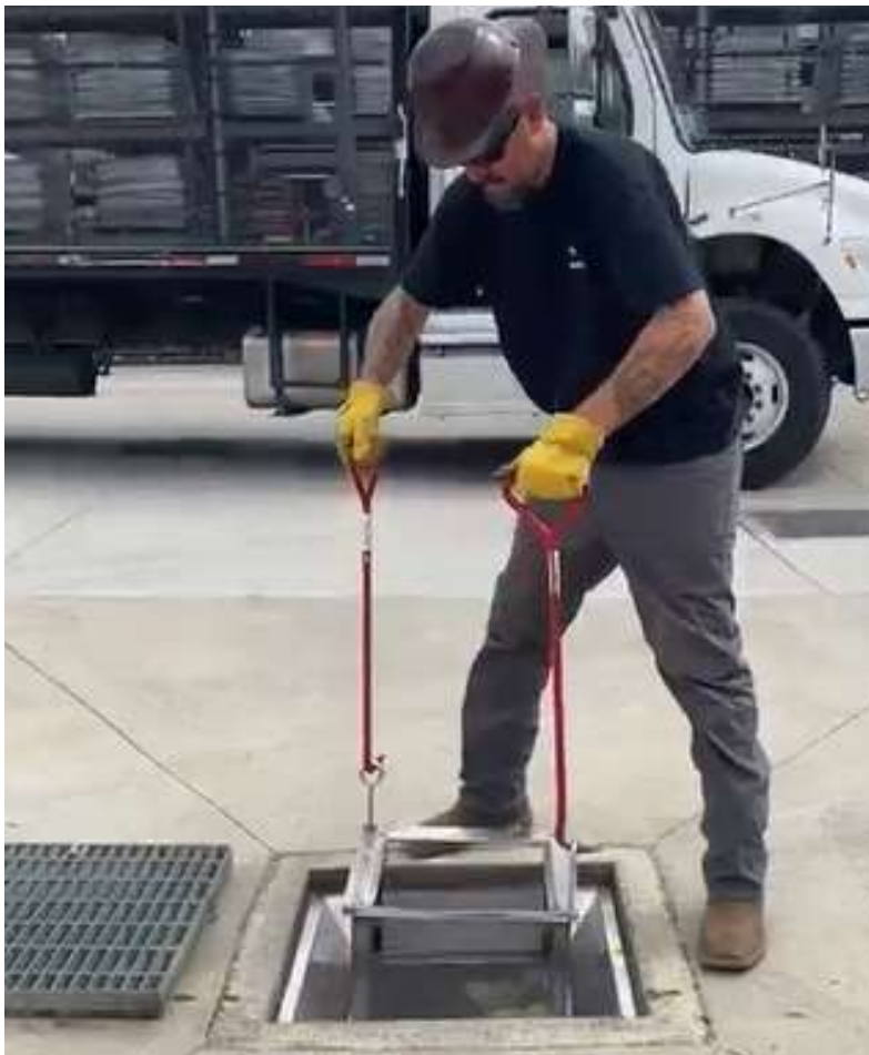
Figure 27 Example of installing the stainless-steel basket within the stainless-steel basket option in a grated inlet (Configuration 1)
