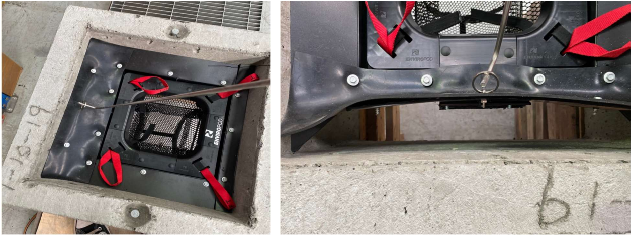
Figure 18 Hinged vector port seal example. For grated inlets (configurations 1, 2 and 3)
