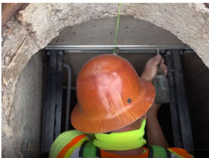
Installation of the LittaTrap Bracket
